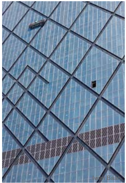
Density of the diagonals varies with the stresses on the buildings.
