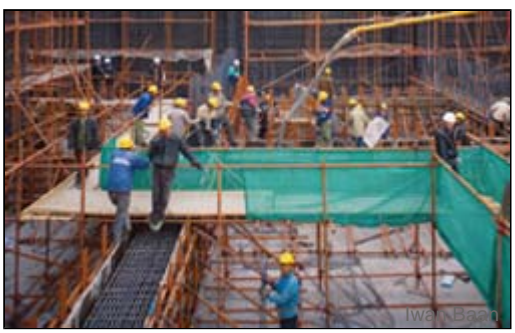
Foundation mat included a record 40,000-cu-m continuous pour that took 50 hours.
